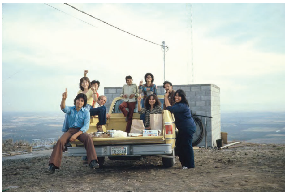
KDNA founders and volunteers building the radio tower on Ahtanum Ridge, 1978-79. Photograph courtesy of Rosa Ramón.
